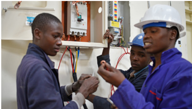
Electrical trainees working on a three phase isolator with a change over switch
