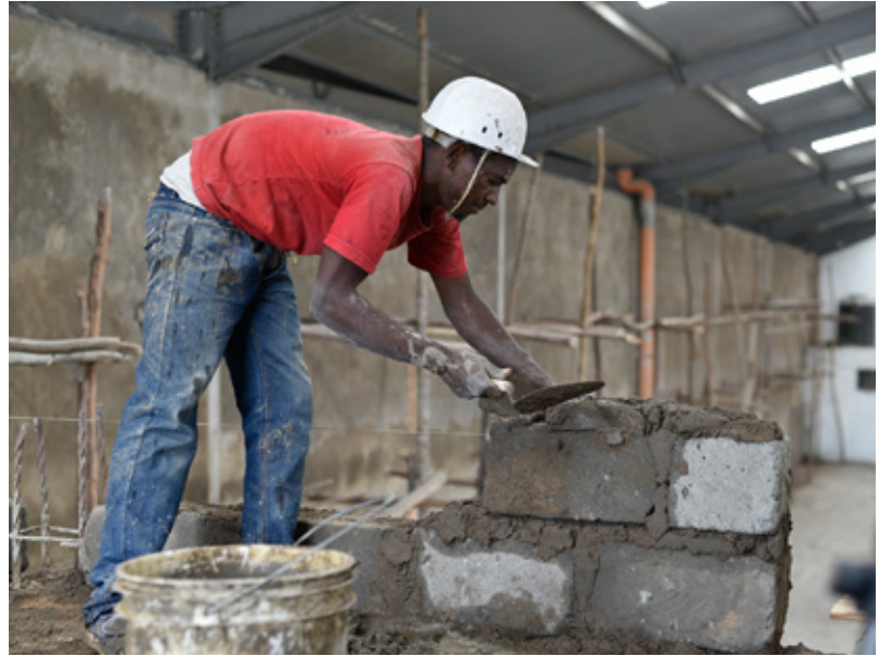
Graduate of CAP YEI in a construction site
