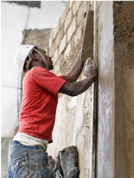
Graduate of CAP YEI in a construction site
