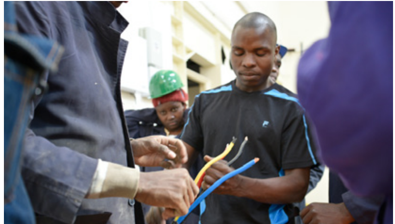
Electrical graduates installing electrical wiring in a construction site
