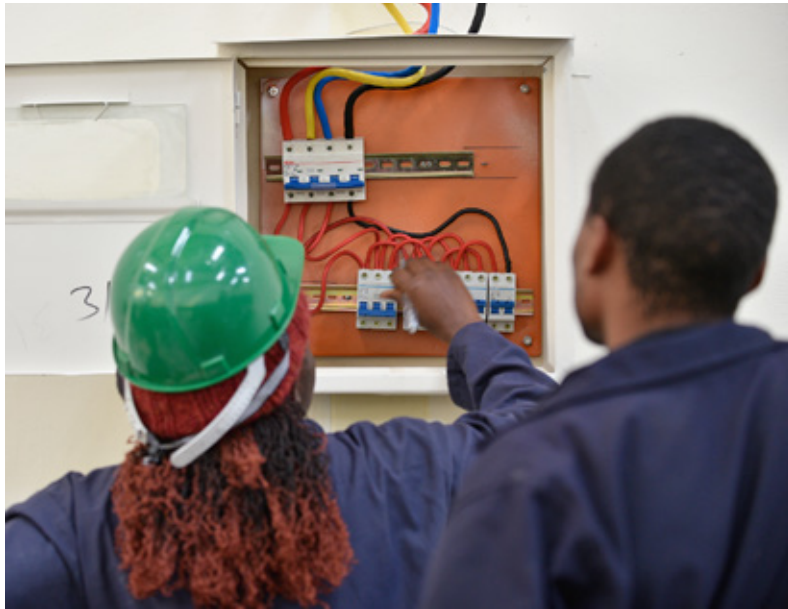
Electrical trainees installing main distribution board circuitry
