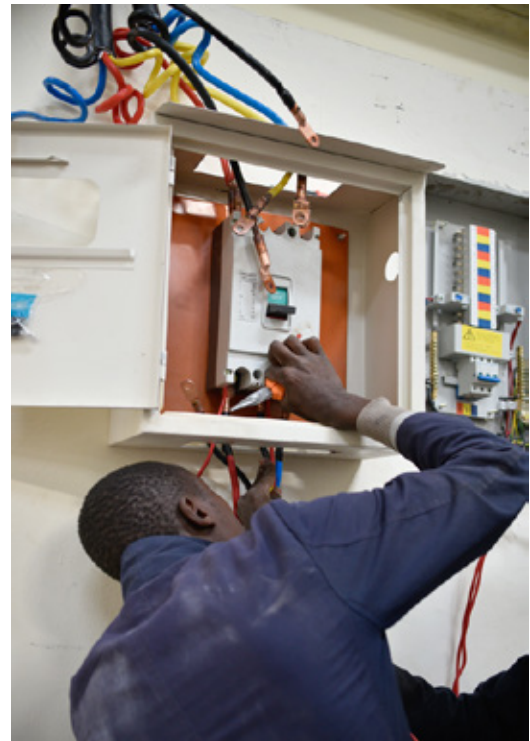
Electrical trainees working on a three phase isolator with a change over switch
